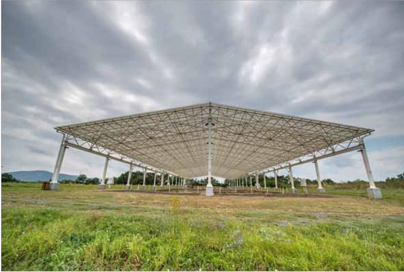
Figure 4. Covering of archaeological site of Selbir part of Gabala city. Photo by SEBA.
